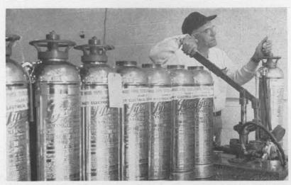
EXERTING 350 lbs. pressure on a five-year-old fire extinguisher, a hydro-static test unit, operated by Jim Schenck (2415), determines if the extinguisher is in safe and efficient operating condition.
